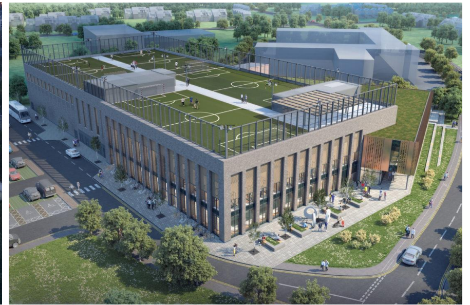
Spelthorne Leisure Centre – ultra energy efficient £1.9m
