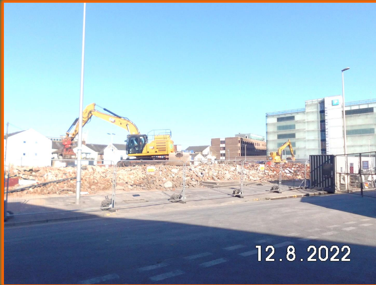
Demolition and Site Clearance of Terraced Buildings 12th August 2022 (Week Minus 25)
