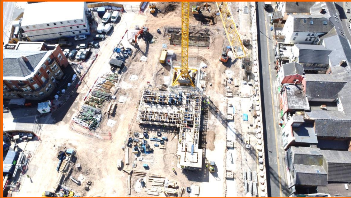
Slip-Form Rig Build 25 th May 2023 (Week 17)
