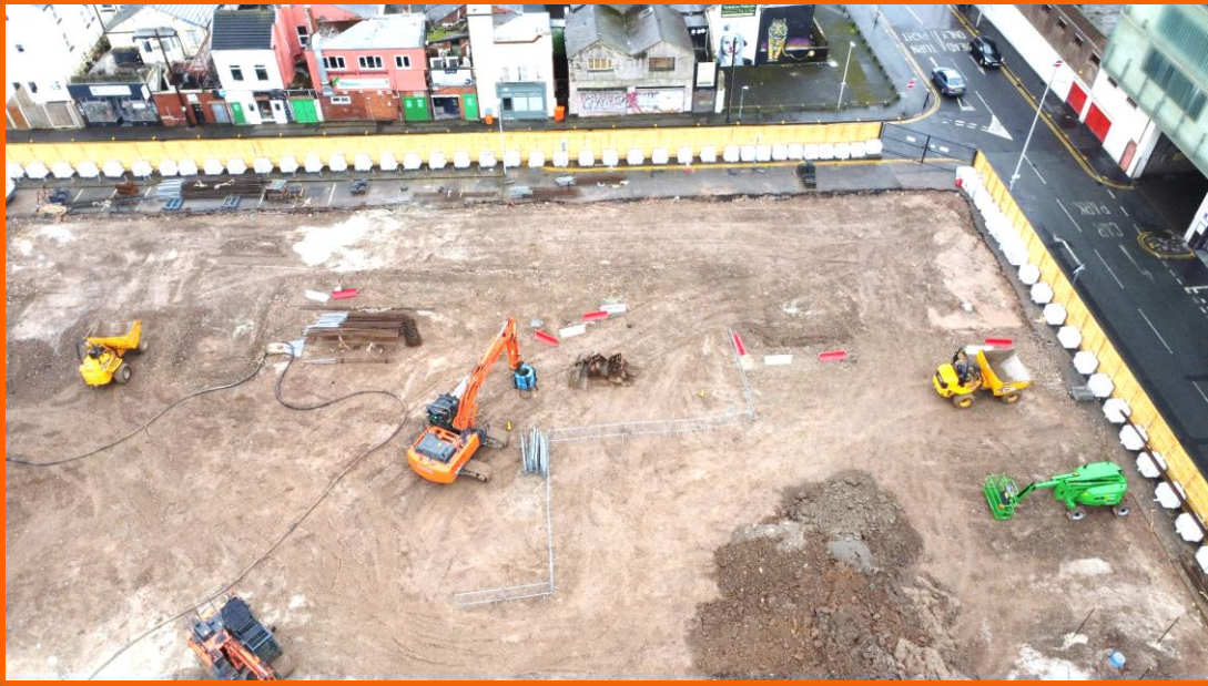
Groundworks Start 29 th March 2023 (Week 9)
