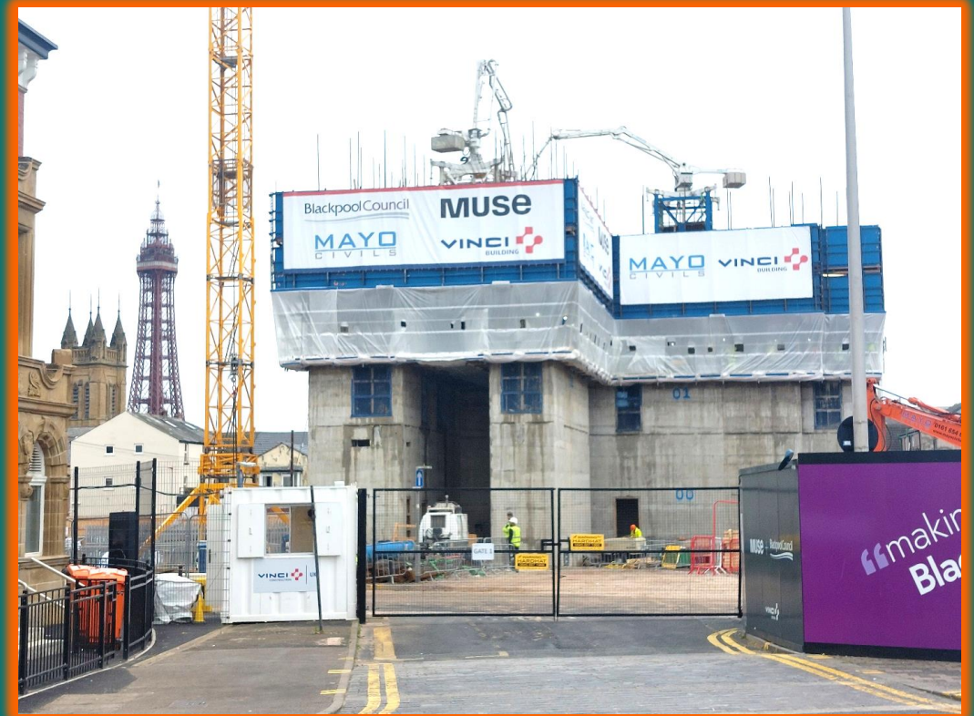
Slip Form Rig Sliding 20 th June 2023 (Week 21)
